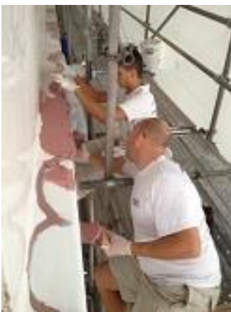
Application fairing in 3 layers
