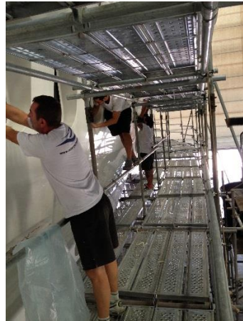
The team work on several deck in the same time
