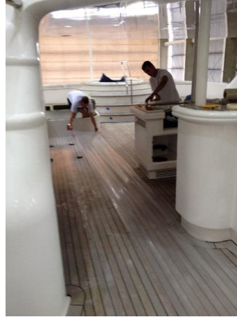
Installation of the protection on the teak
