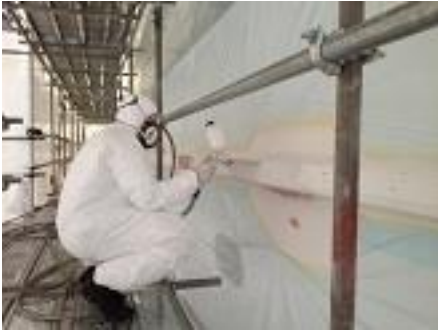
Ultra Build application by spray
