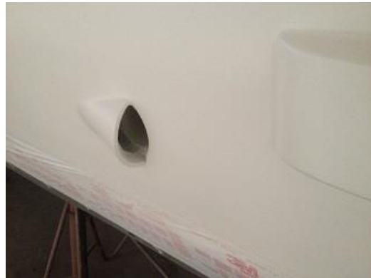
With coating of 545 in two layers
