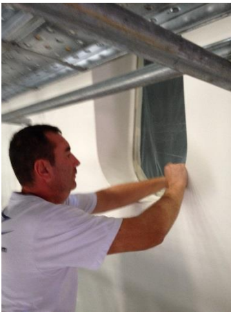
Porthole taping protection
